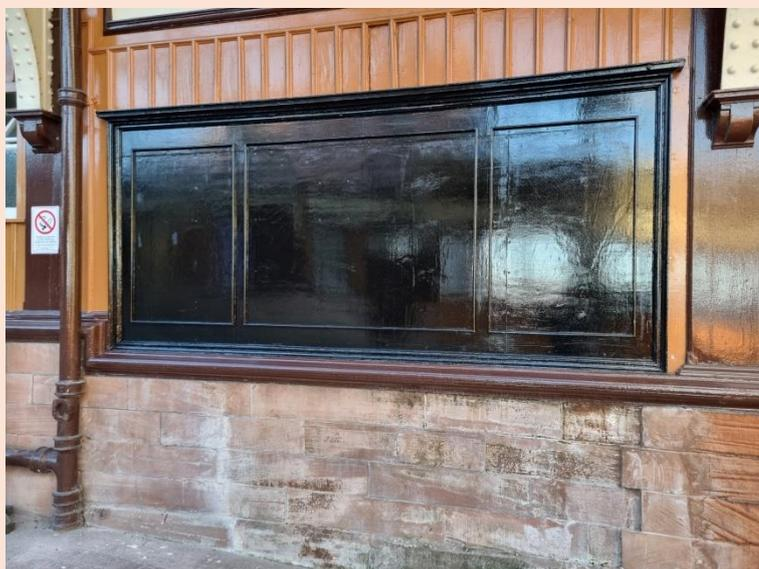
**Left:** The finished job, with all of the rotten wood replaced and the poster board awaiting Leo's art work.
